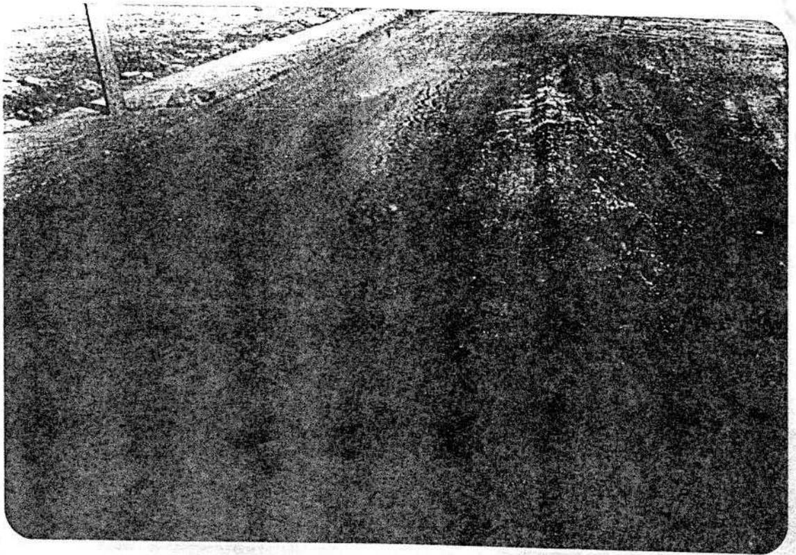
Fig. 3 : Initiation of pavement disintegration in an affected area.
