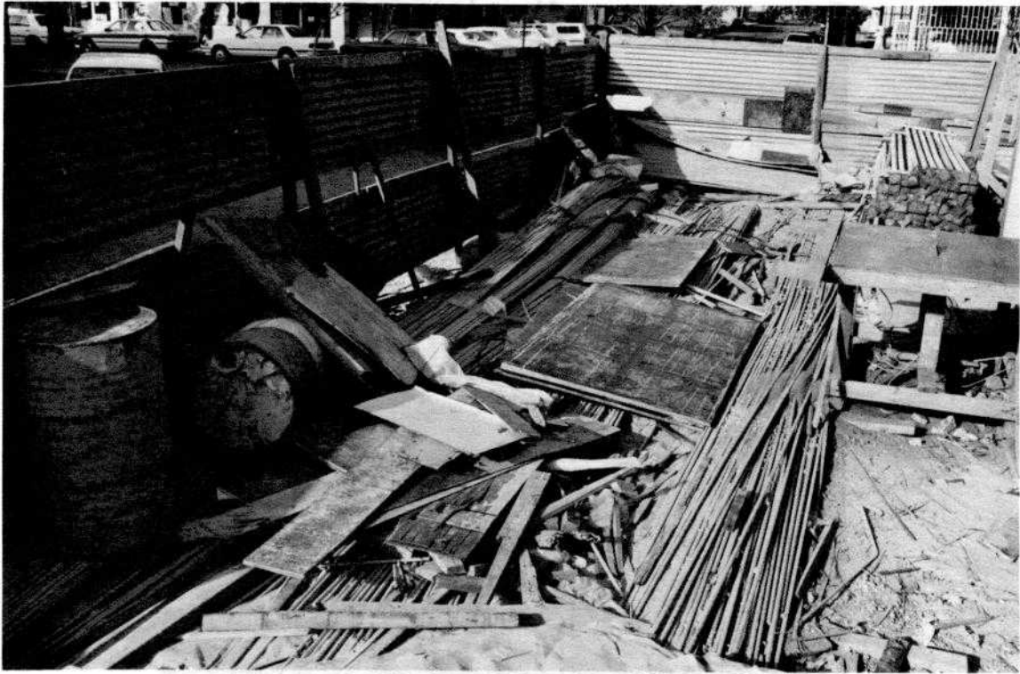
Fig. 5. Storage of FBECR at construction site
