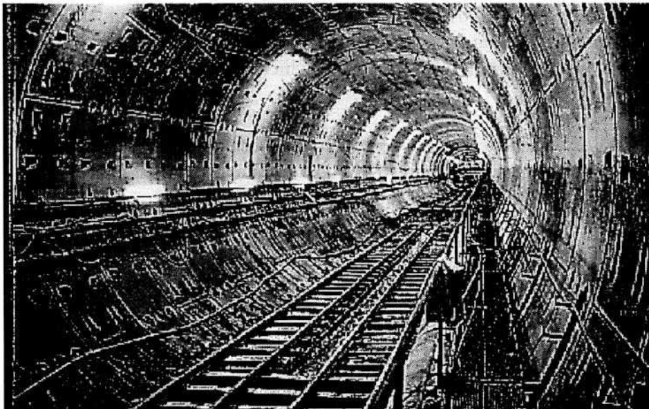
Figure 10: Bored railway tunnel lined with precast concrete segments.
