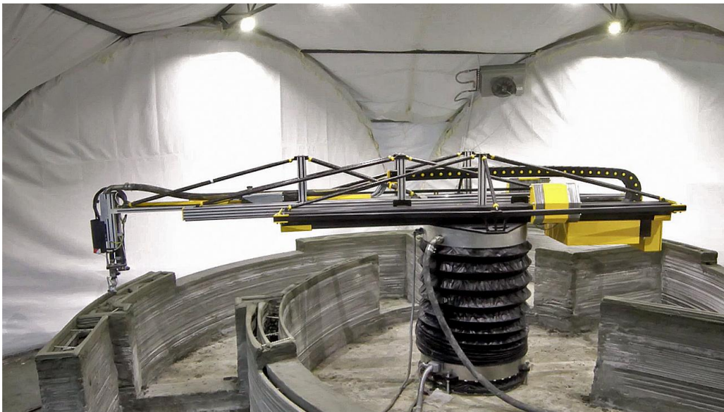
Figure 2.12: Stationary rotational robotic system developed by ApsiCor Source: (Dörfler, 2018)
