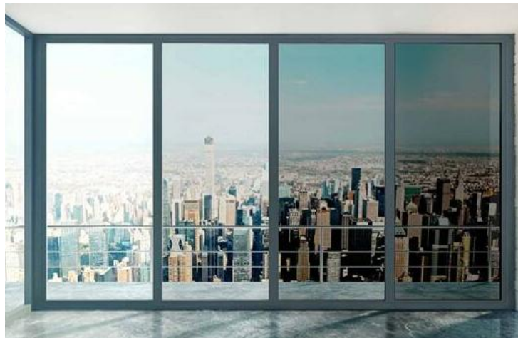
Figure 5: Tinting states of electrochromic (EC) glazing
