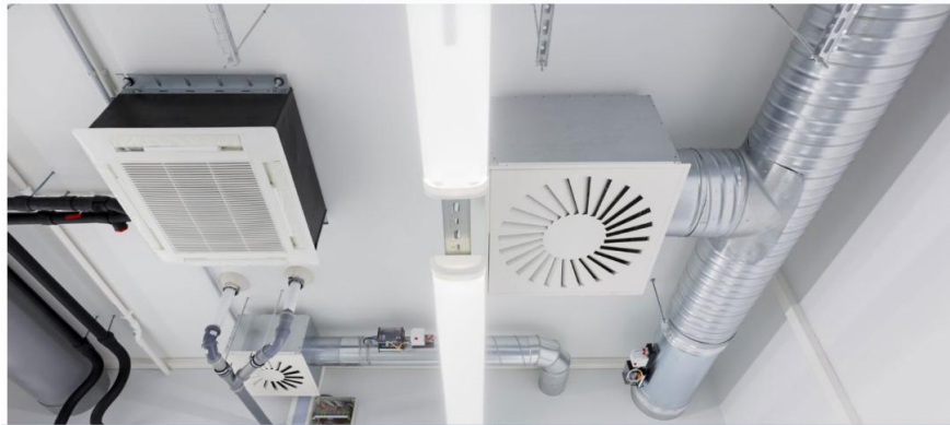
Figure 6: Multi-port Supply ventilation system
