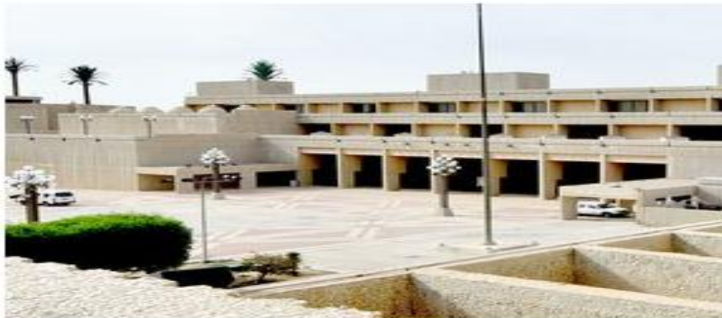
Figure 23: College of Design & Built Environment (Building 19) KFUPM
