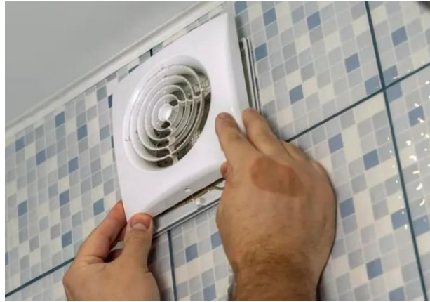
Figure 4: Extractor fan hung on a tiled wall Source: Forbes.com
