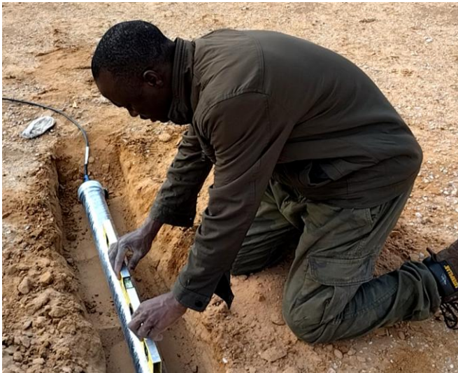
Figure 4.8 Leveling and fixing the cable.
