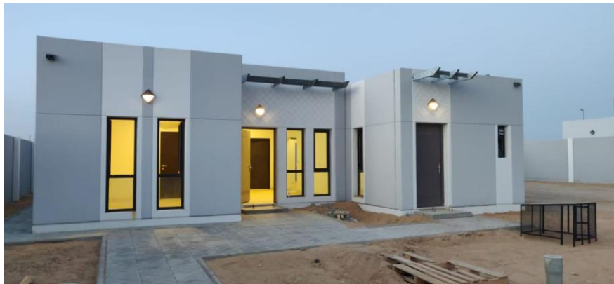
Figure 4.10.4 The Rabigh Developmental Housing Project-Project D
