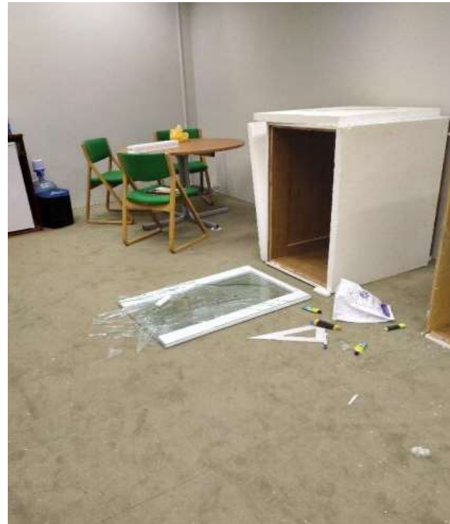
Failed trails- Glass structural failure
