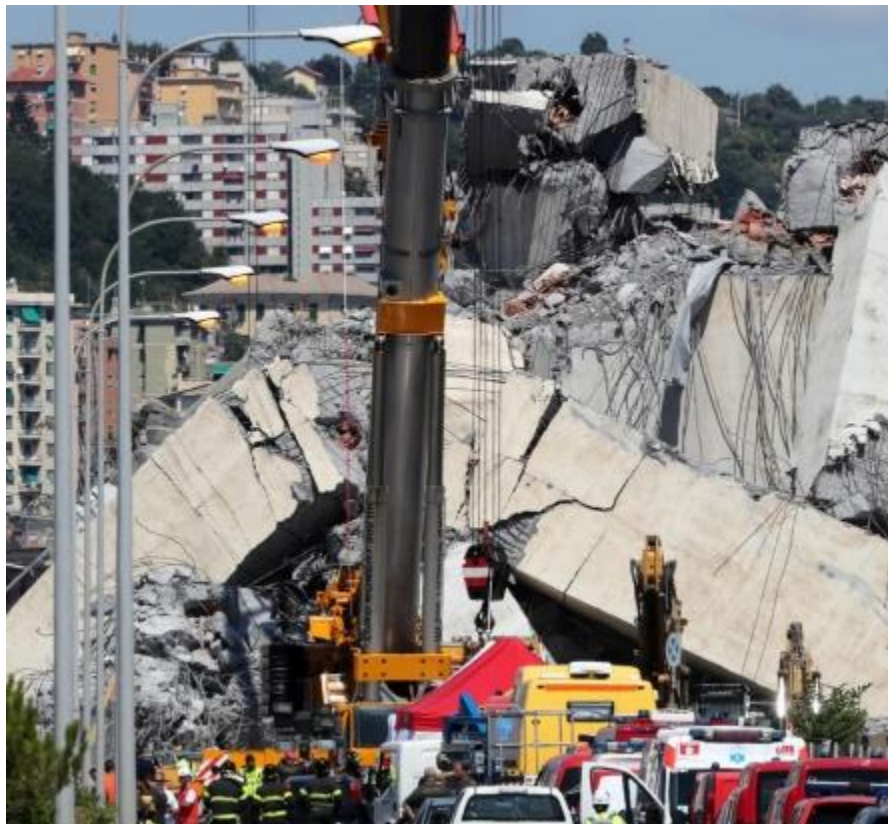
Figure 1 The collapse of Genoa Bridge in 2018. Corrosion was one of the major factors of the disaster [32]. Adopted from [33]
