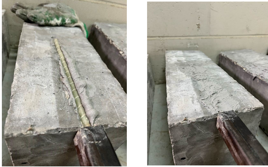
Figure 16: Installation of FRP bars/strips
