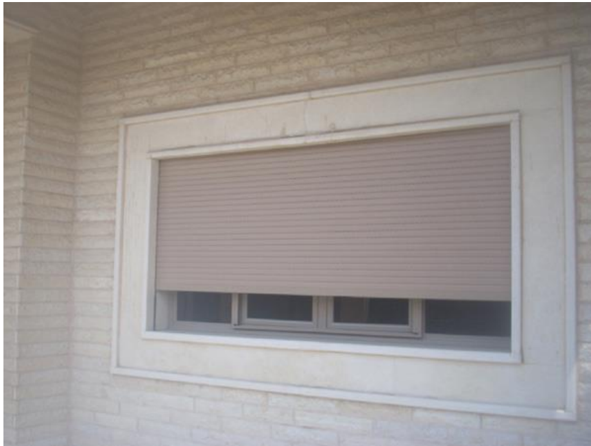
Figure 2.20 A widely used window shutter to block the heat flow into residential buildings [130].
