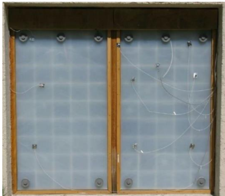
Figure 2.27 External view of the PCM-aerogel passive solar wall [166].
