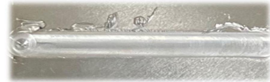
Figure 16e: Surface appearance joint #5
