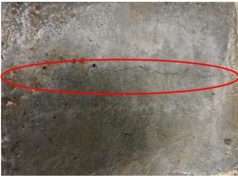
Figure 4. 11: Crack appearance of 0.25mA/cm 2 Specimen
