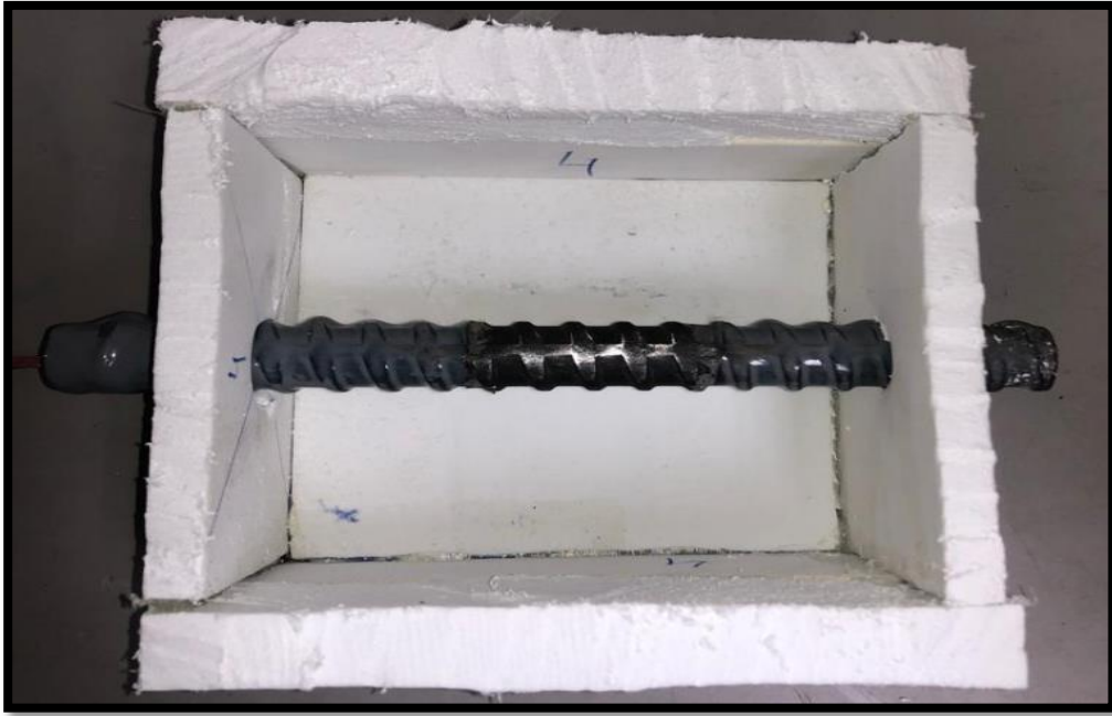
Figure 3. 8: Before casting concrete, embedded Steel bar along FBG sensor.
