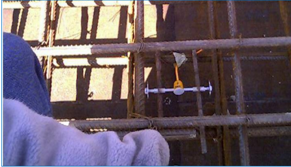
Figure 2. 15: Installation of VW strain gauge [57]
