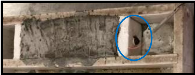
Figure 3. 4: Fiber optic test after 24 hours of concrete casting
