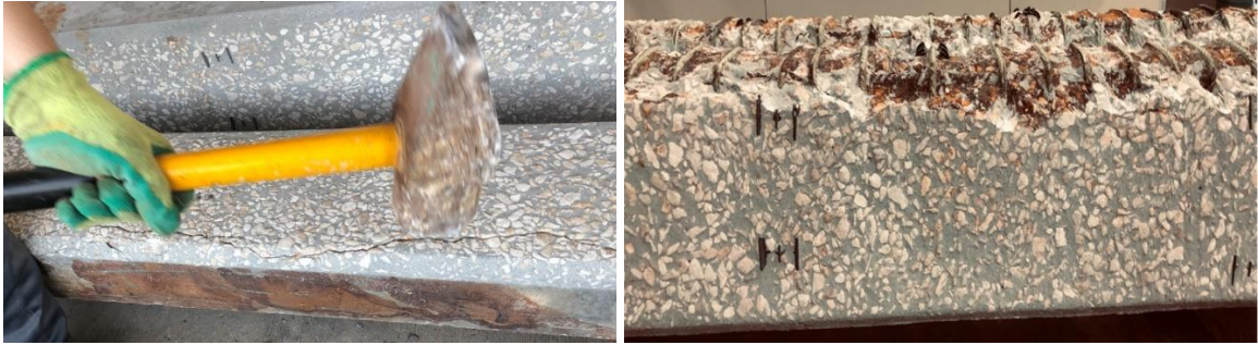
Figure 3.23: Remove concrete cover and cleaning the corroded bars
