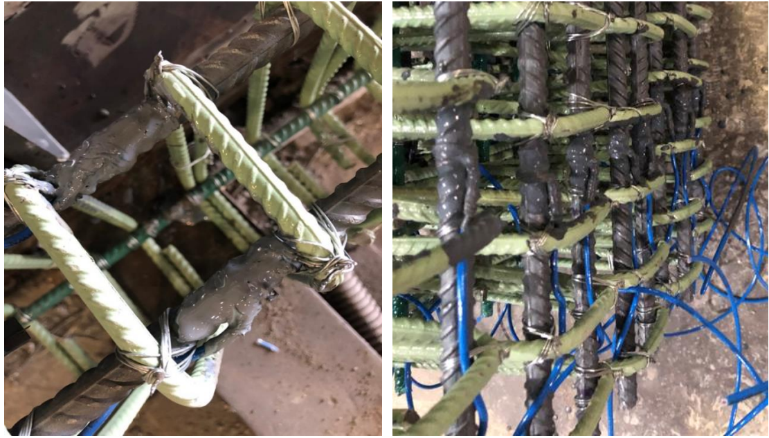
Figure 3.4: Applying an epoxy coating to the connection portion.
