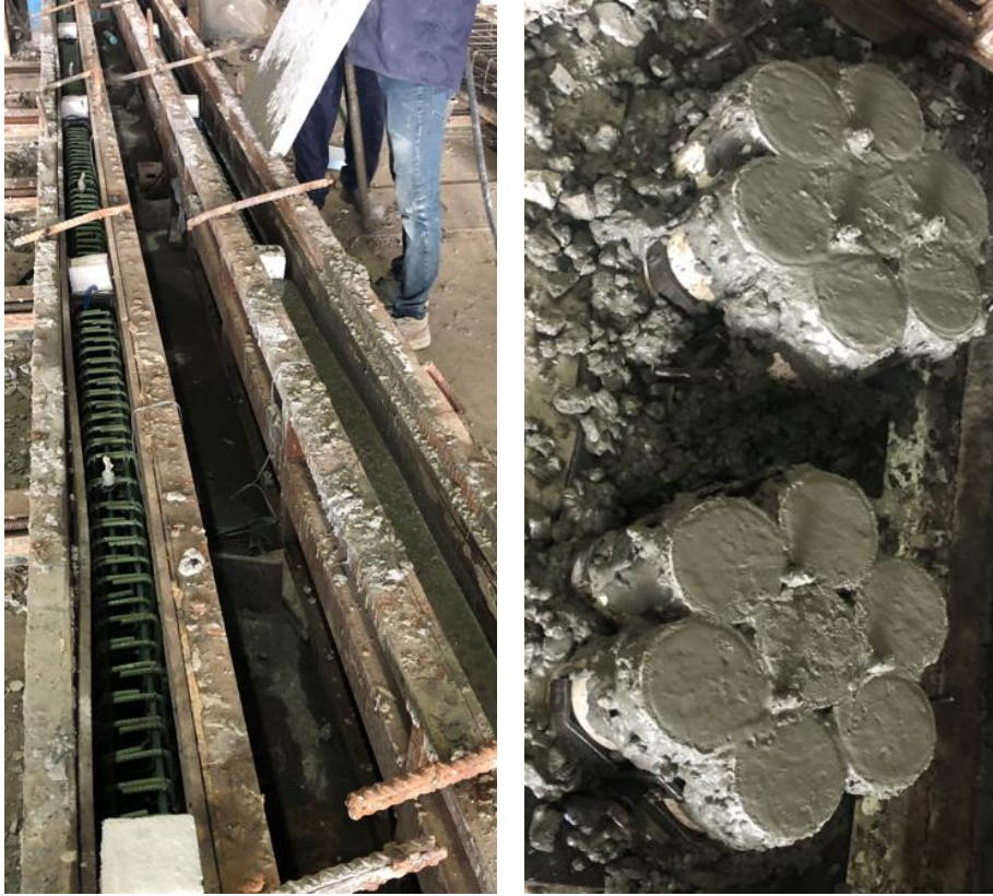
Figure 3.5: Concrete casting (a) Casting of beam Specimens (b) Casting of cylinders.
