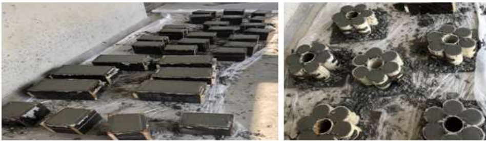
(e) Casting of the concrete substrates into different molds
