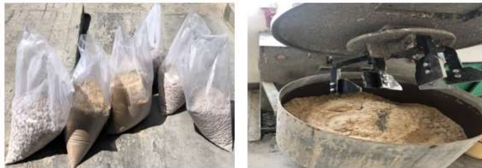
(a) Preparing and mixing the materials
