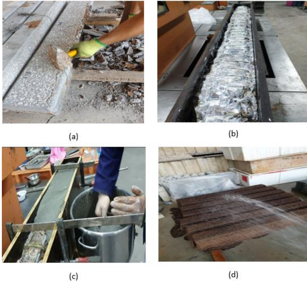
Figure 35: (a) Cover removal. (b) Bonding agent application. (c) Repair material placement. (d) Water curing.
