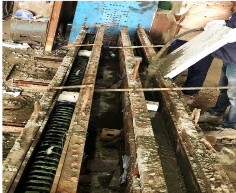
Figure 20: Casting of the beam Specimens.
