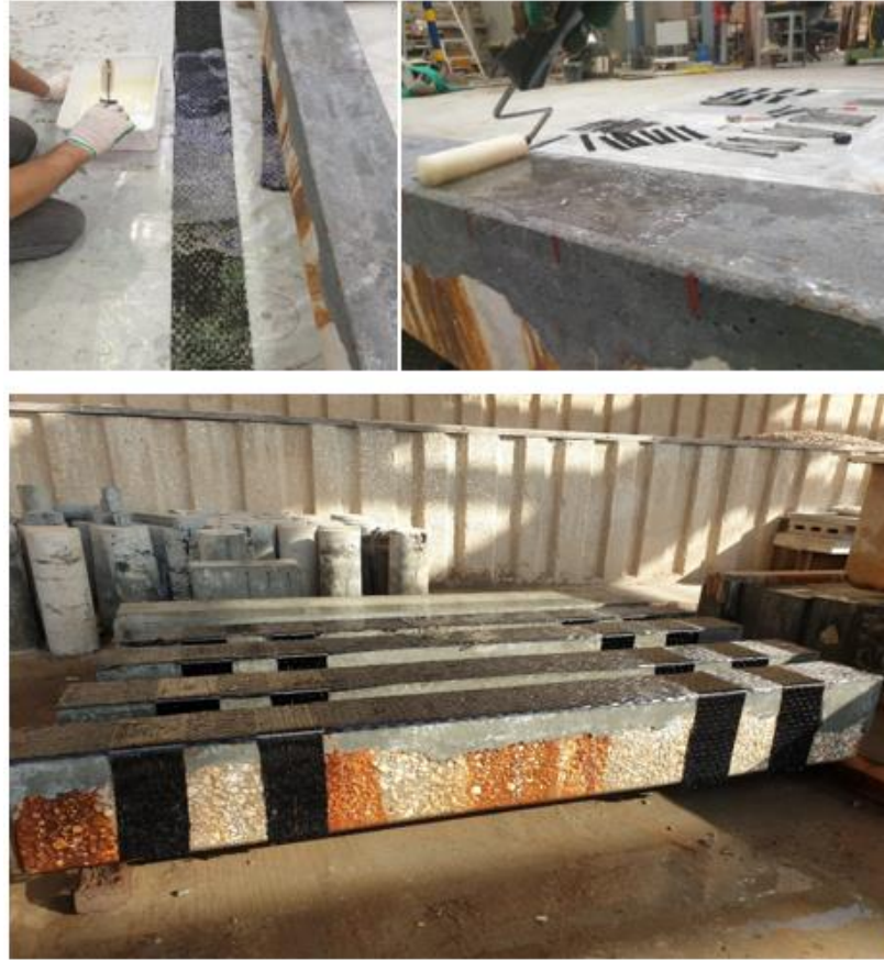
Figure 37: CFRP work
