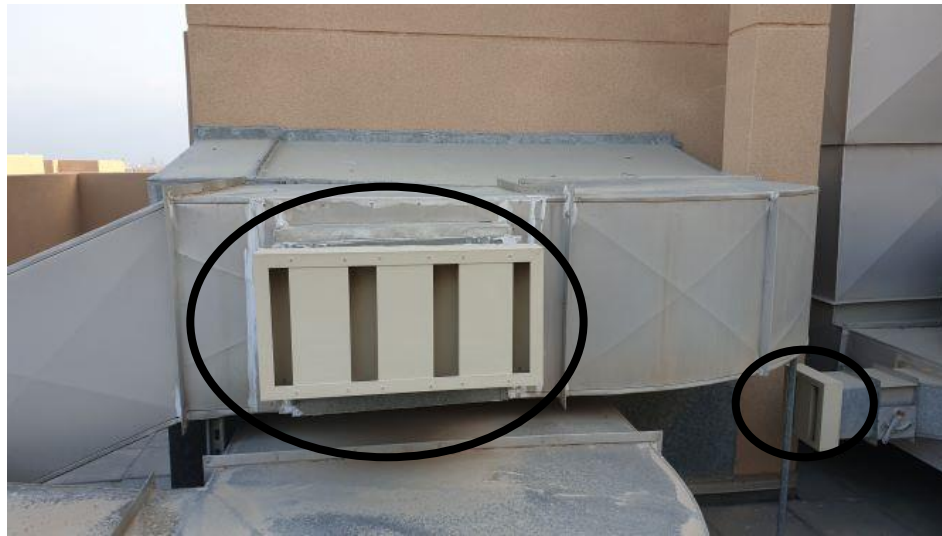
Figure 3.5: Outdoor air inlets
