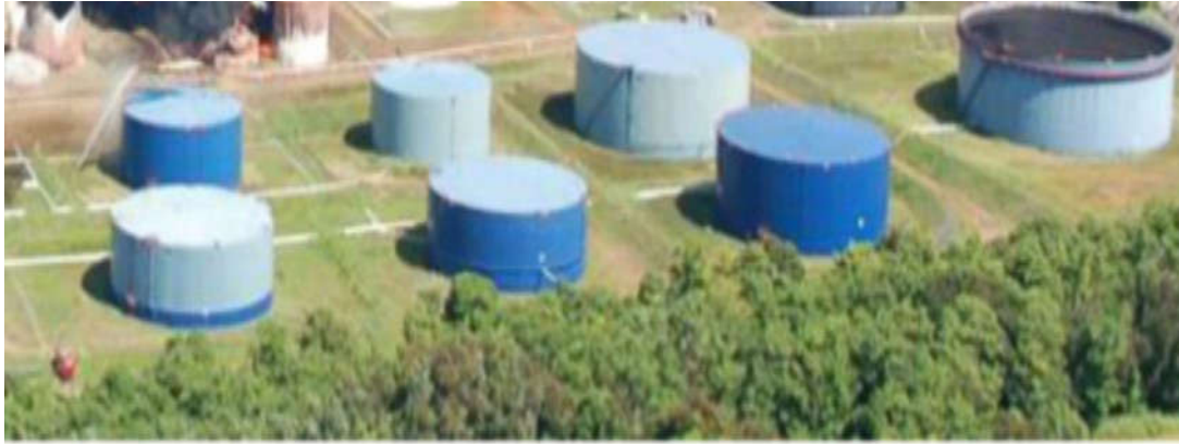
Figure 1 Cylindrical tanks in an oil field [1]
