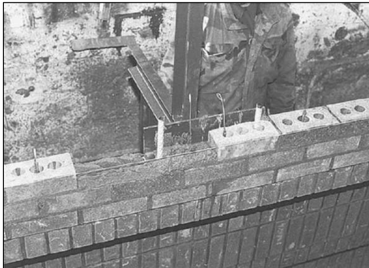
Figure 2.13: Construction of prefabricated brick panels by masons
