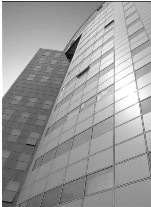
Figure 2.9: Prefabricated metal panels
