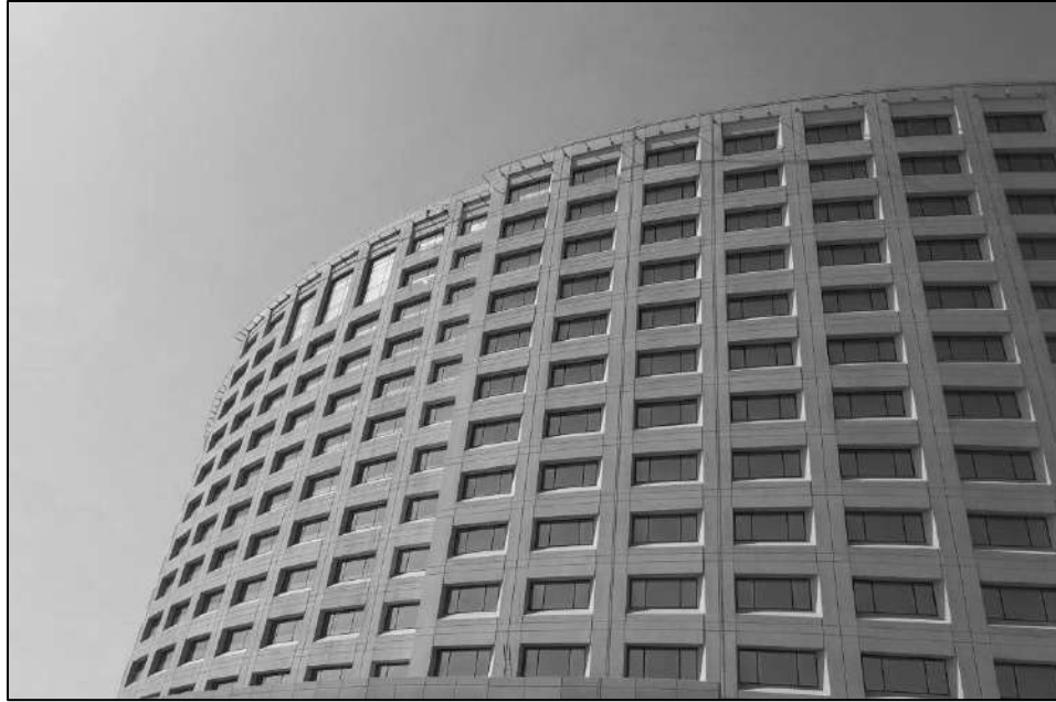
Figure 2.11: Precast concrete wall panels
