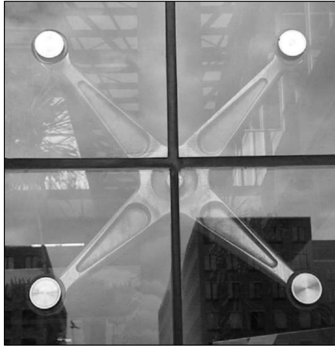
Figure 5: Spiders fixed to building frames are used in structural standoff systems (Spider System)
