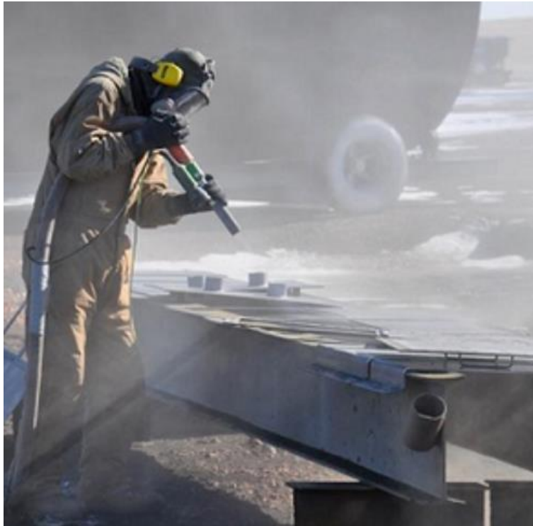
Figure 3.4 Abrasive blasting in progress
