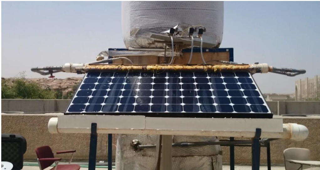
Figure 5-16 : Front view of PV cooling system control using ON-OFF valve
