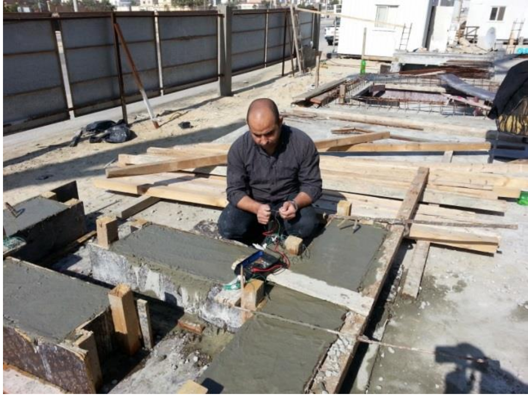
Figure 4.23: Checking the voltage of wire after casting
