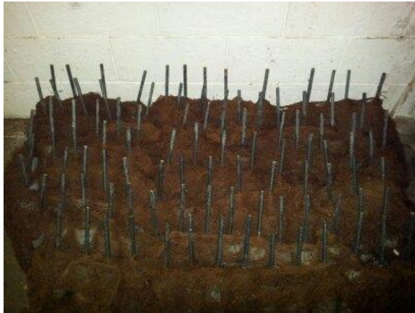
Figure 3.7 Curing Using Wetted Burlap.
