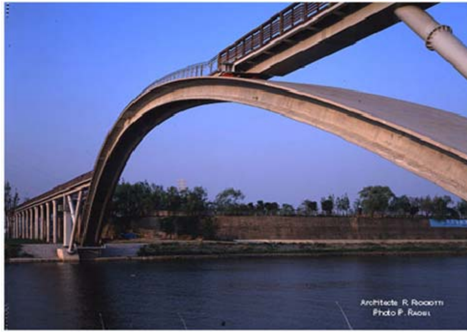
Figure 1.6: Seonyu footbridge, Korea, 2003 (8th Hitachi EU Science and Technology Forum, Athens, May 20-22, 2005) Arch span 120 m deck thickness 3 cm.
