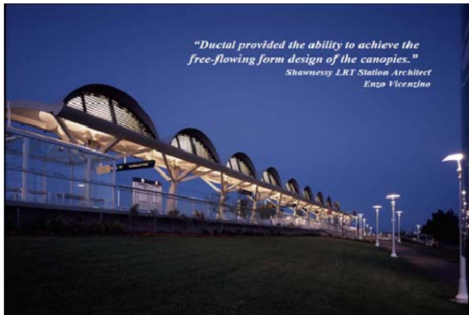
Figure 1.7: LRT Train Station, Shawnessy, Canada, 2003 (Images from Lafarge) Canopies 5×6 m, 2 cm thick, supported on single columns.
