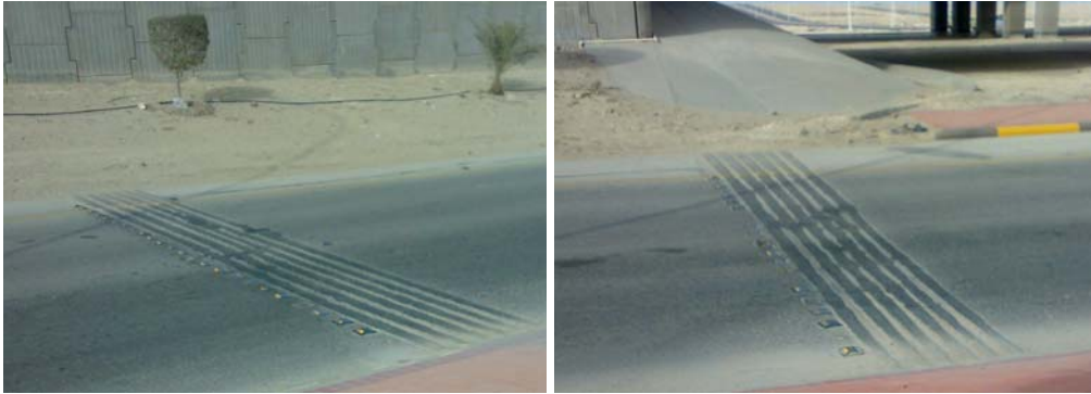
Figure 1.2: Short periodic humps at Dammam-Dhahran highway and Doha.
