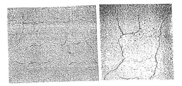
Fig. 5. Shrinkage cracking in deck slab
