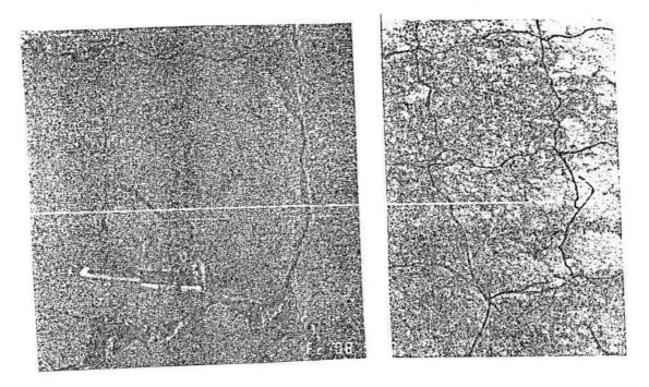
Fig. 3. Stress induced cracking at soffit of deck slab
